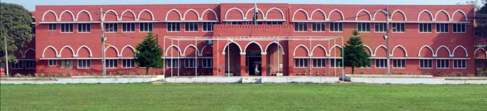
Front view of the Main Block
