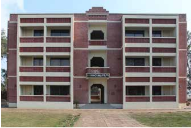
Shah Navaz Mallick Block (Teachers' Residence)
